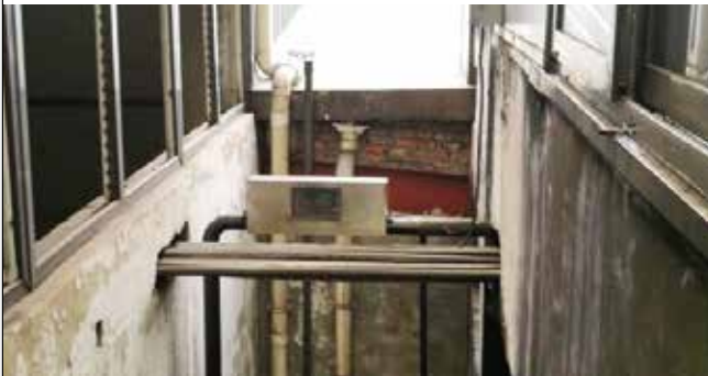
Vulcan S25 outdoor installation
