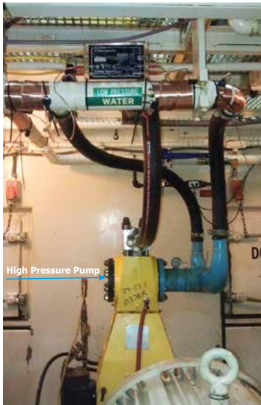
Vulcan S25 was installed on the high pressure wash station in the Chrysler ITP 2 plant.
