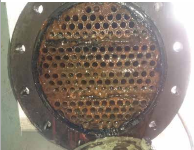
Heat exchanger before Vulcan installation
