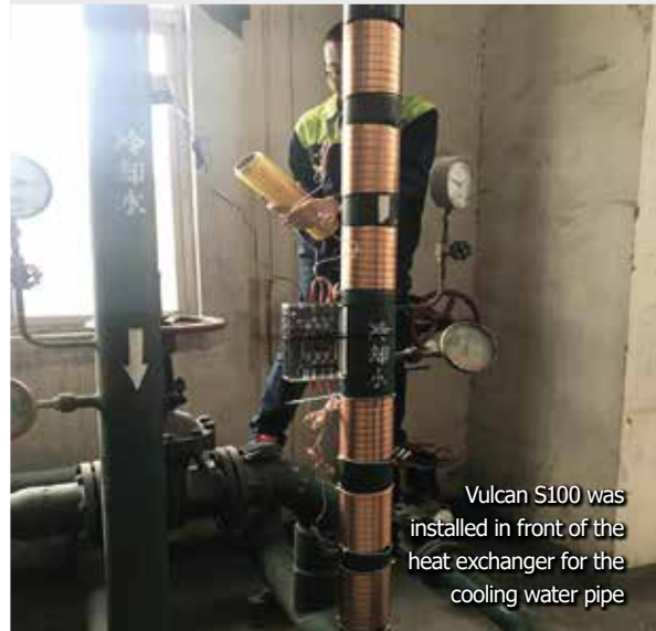
Vulcan S25 was installed in front of the heat exchanger for the cooling water pipe
