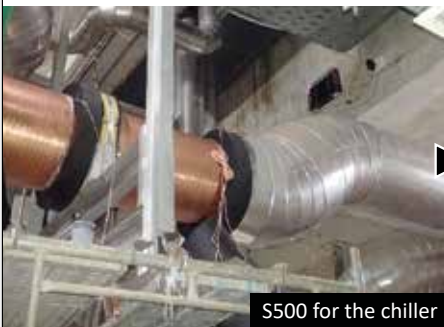
Impulse bands covered by pipe insulation
